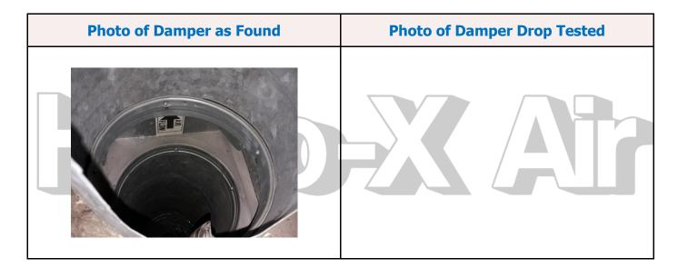
Due to the size of the damper it was not possible to drop test, recommend replacing to externally testing fire damper.
